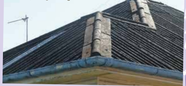
Super six roofing ridge capping and guttering
