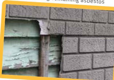
External cladding containing asbestos
