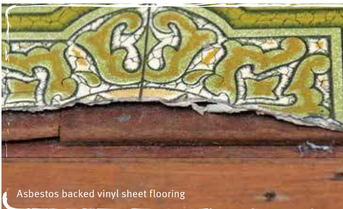
Asbestos backed vinyl sheet flooring
